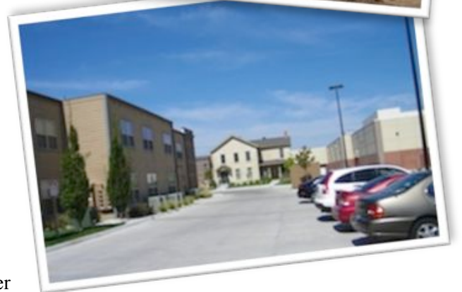
Pictured at top is an orphaned Strasser House in 2009, its surrounding neighborhood demolished. Below, the Strasser House in its 2012 neighborhood.
