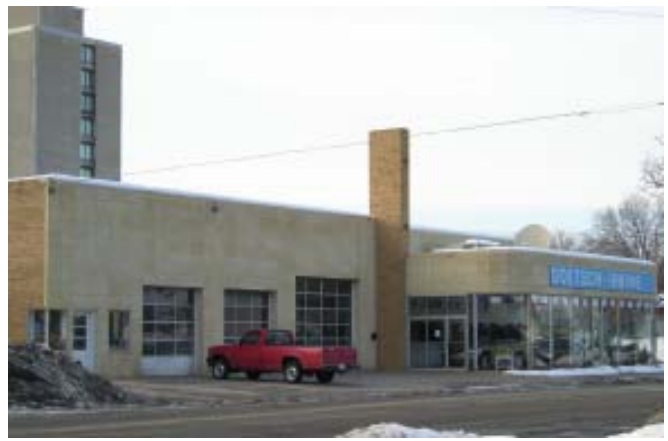
Goetsch-Irvine Building, 221 North 4th
