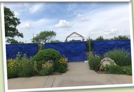
Top, the conservatory in 2022. Bottom, demolition in progress in May 2023.
