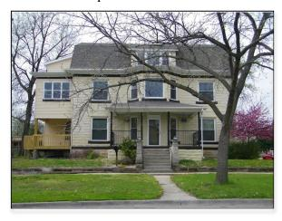
Constructed of formed concrete blocks in 1905, the house was in need of many repairs. The owners stabilized the foundation, repaired exterior cracks, rebuilt the side porch, added a new roof, new wiring, and new plumbing, and completely updated the interior.
