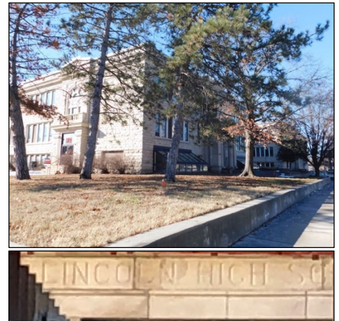
Top, the newly renamed Lincoln Education Center. Bottom, a close-up of the "Lincoln High School" lettering partially visible past the ongoing renovations.
