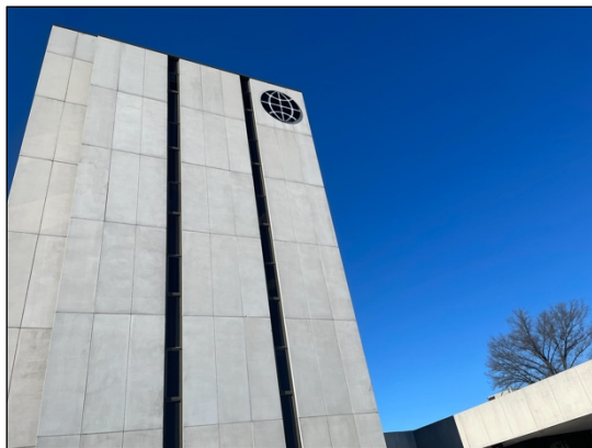
Above, detail view of the east tower elevation.
