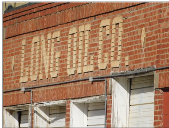
Top, a vintage photo of the Long Oil station at Fifth Street and Poyntz Avenue. The photo is courtesy of the Riley County Historical Society and Museum. Bottom, a close-up of the brick Long Oil Company sign on the garages at 621 South Juliette Avenue.
