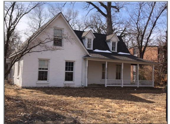
Above, 721 Pierre Street in February 2023.
