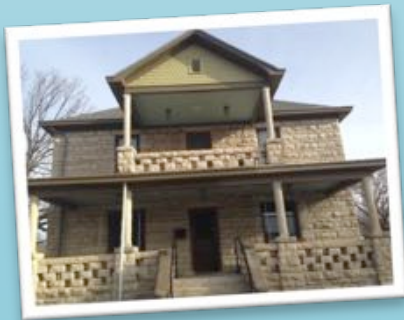
Above, 720 Poyntz Avenue, which was recognized with a Historic Preservation Building Award in 2015.
