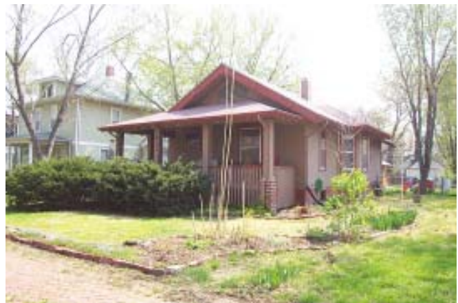
Above, 811 Osage, belonging to Sara Fisher. She spoke in favor of the TNO District before the Commission on February 9, 2004, saying that she is in the process of converting her property back to a single-family house.
