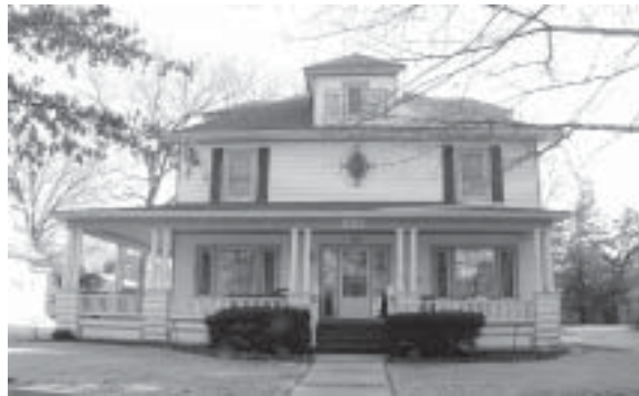
825 Pierre The Amy and Frank Gatschet home. Built in 1910 by the West family who ran the “inter-urban” streetcar line from here to Junction City.
